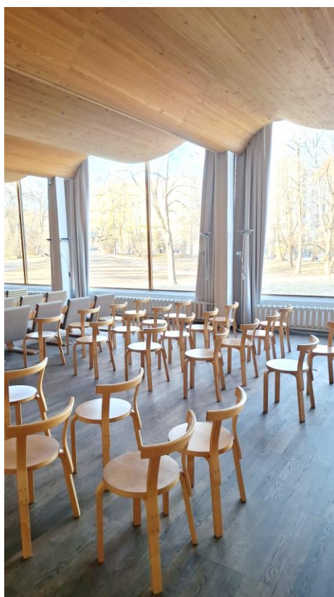
Figure 4. The wave ceiling of the lecture hall of the Alvar Aalto Library in Vyborg (architect Alvar Aalto, 1935). The restoration of the lecture hall with the suspended wooden undulating ceiling took place between 2006 and 2009. The ceiling was recreated according to the original Finnish drawings (The Finnish Committee, 2009). – Photo by Olga Erofeeva.
